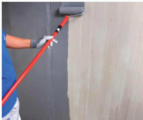
Application of Eco Prim Grip Plus on concrete by roller
