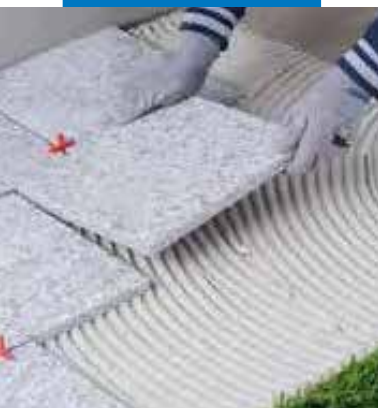
Installation of natural stone in exterior
