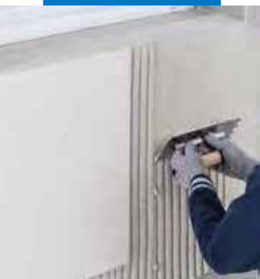
Installation of large-size ceramic tiles
